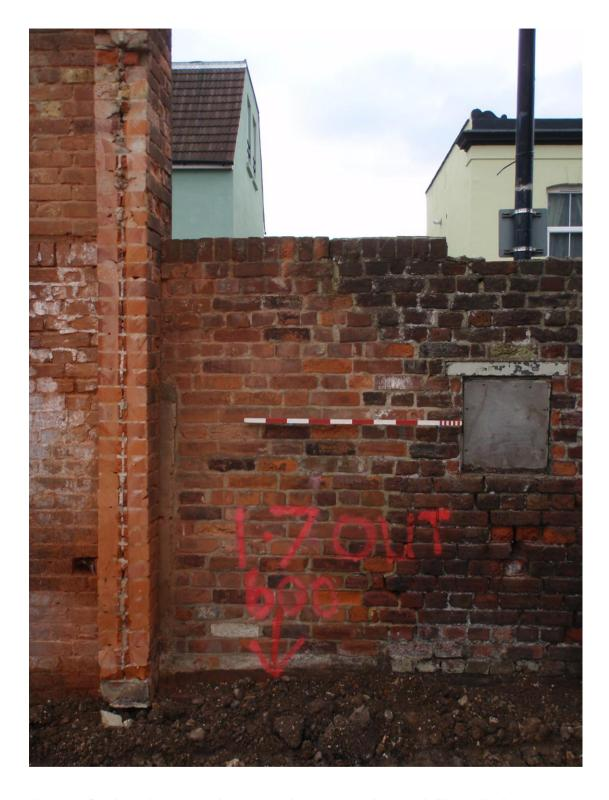
Plate 12. Section of wall showing small window and brick repair [W04, W07]
